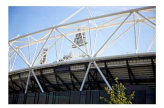
Rogers style, with its operating plant (such as air conditioning) sited on the outside of the building to reduce the heat inside.
